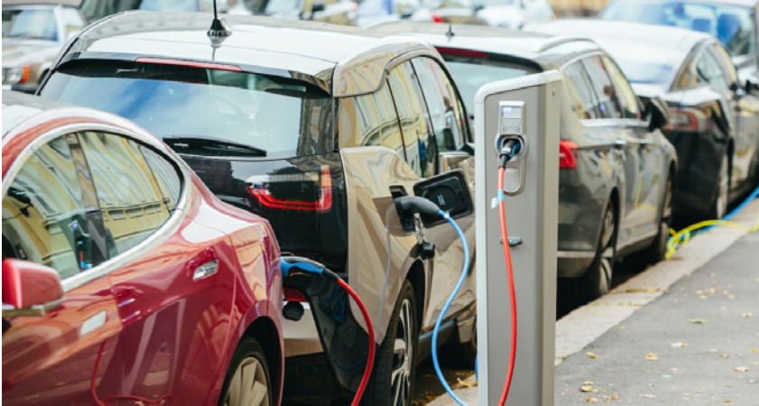
Europe is failing to deliver the infrastructure required for the clean mobility revolution.
